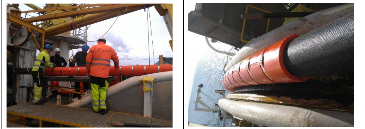
Figure 29 Installation of PPLDUCT on cable
