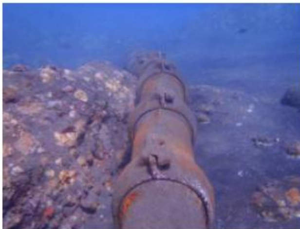
Figure 3-2: Cast Iron Shells Enclosing a Cable
